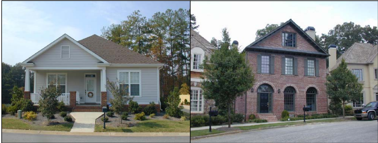
Figure 7.21: Reduced Side Yard Setbacks and Narrower Frontages Used on Residential Development Sites
