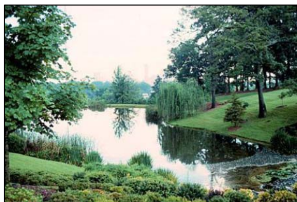
Figure 8.1: Stormwater Pond (Source: Atlanta Regional Commission, 2001)
