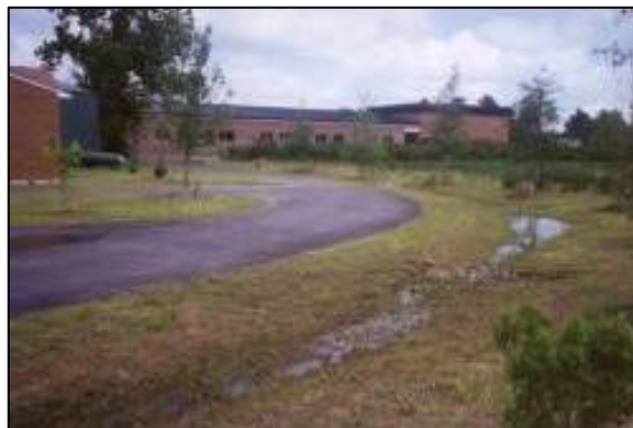
Figure 8.5: Wet Swale (Source: Center for Watershed Protection)
