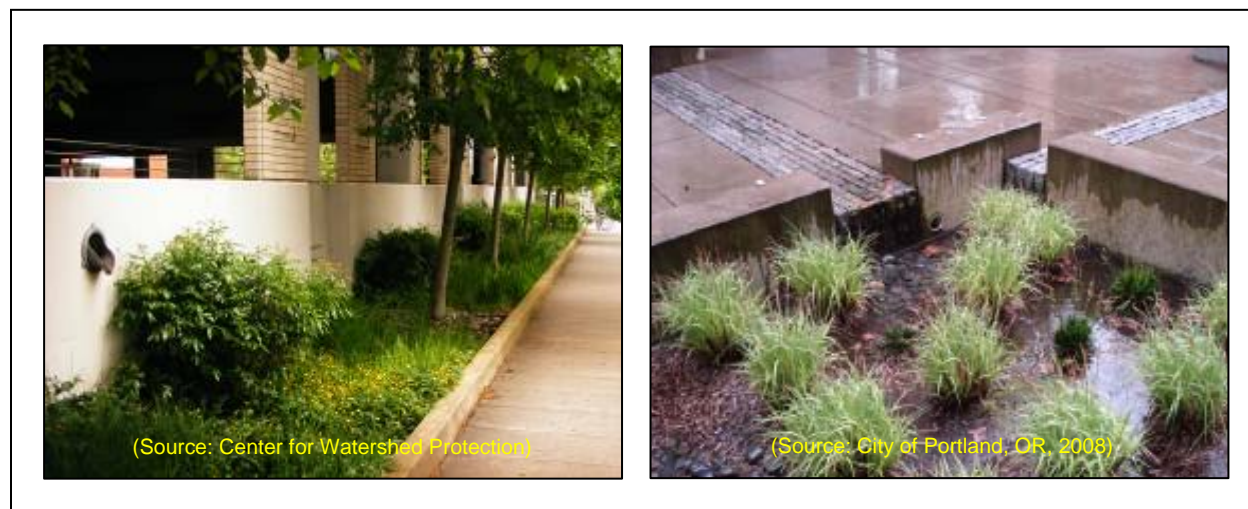
Figure 7.38: Various Stormwater Planters
