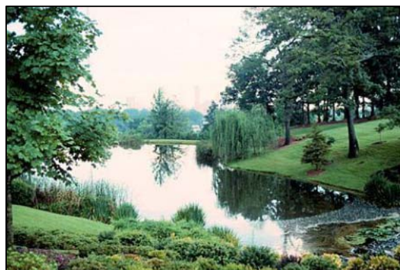
Figure 6.15: Stormwater Pond (Source: Atlanta Regional Commission, 2001)
