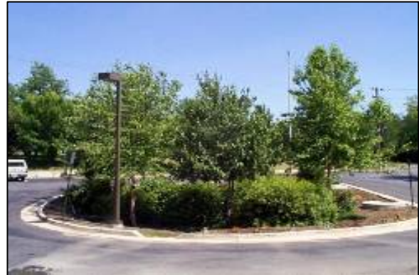
Figure 8.3: Bioretention Area (Source: Center for Watershed Protection)
