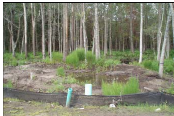
Figure 3.11: Excessive Sediment Accumulation in a Freshwater Wetland
