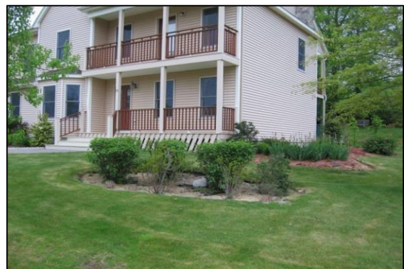
Figure 7.3: Rain Garden Used to “Receive” Stormwater Runoff
