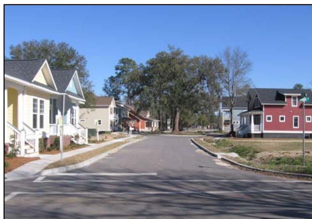
Figure 7.18: Residential Development Site with Sidewalks on One Side of the Street (Source: Center for Watershed Protection)
