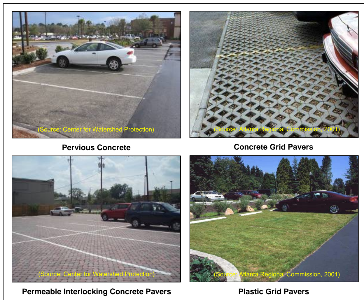
Figure 7.29: Various Permeable Pavement Surfaces
