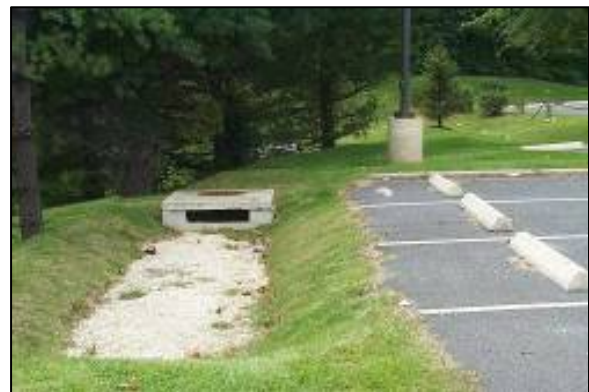
Figure 6.18: Infiltration Trench (Source: Center for Watershed Protection)
