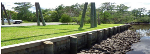
Rip Rap Bank
