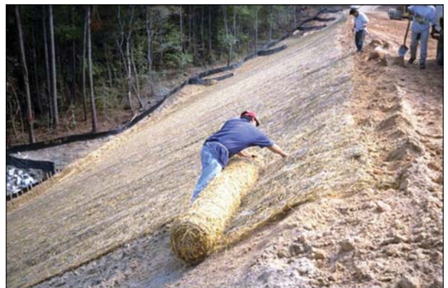
Figure 2. Installation of Jute Matting
