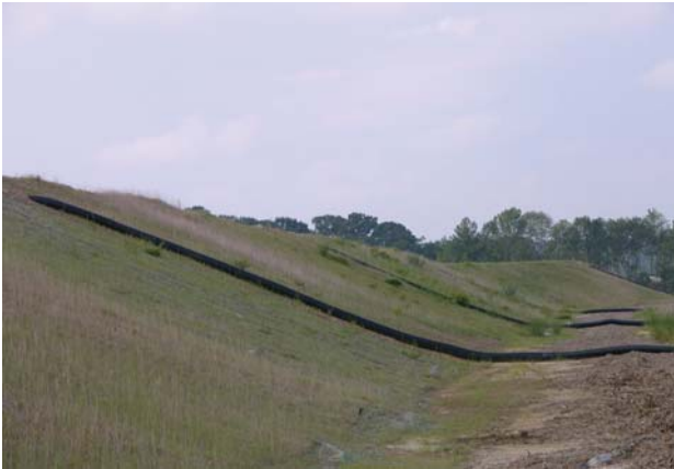
Figure 2. Diagonally Placed Downdrain
