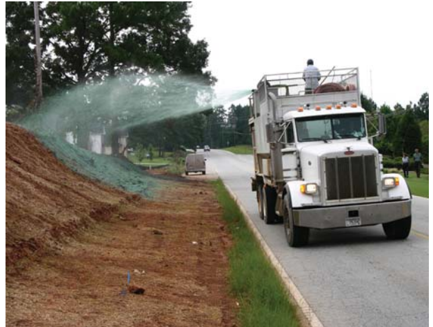
Figure 1. Hydroseeding on disturbed areas
