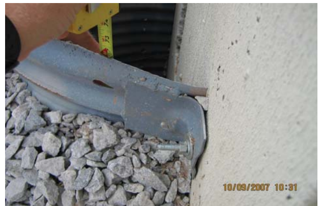
Figure 2. Affixed to Concrete Structure
