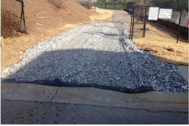
Figure 2. Geotextile Underliner
