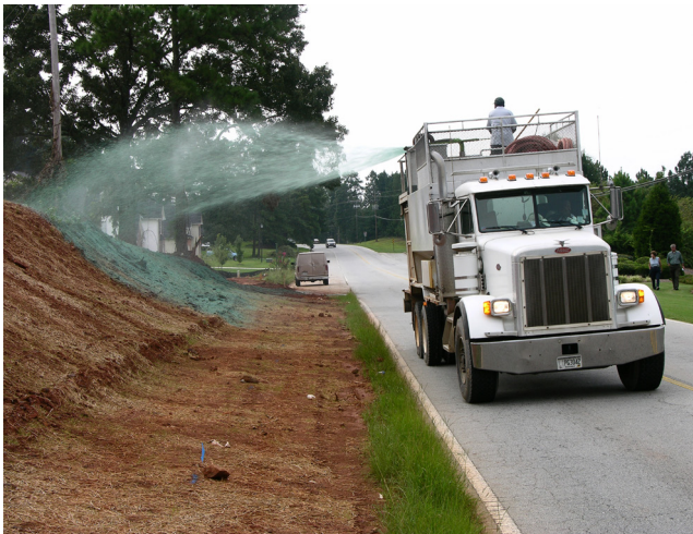
Figure 1. Hydroseeding on disturbed areas
