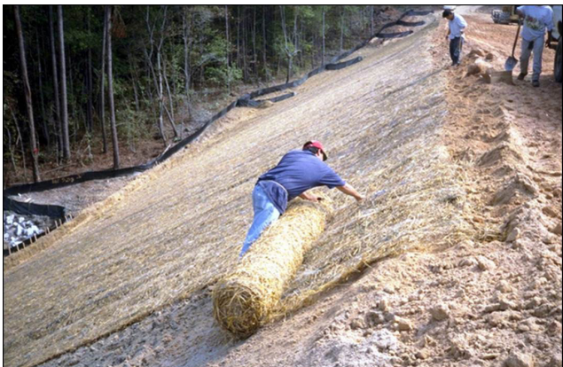
Figure 2. Installation of Jute Matting
