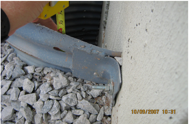
Figure 2. Affixed to Concrete Structure
