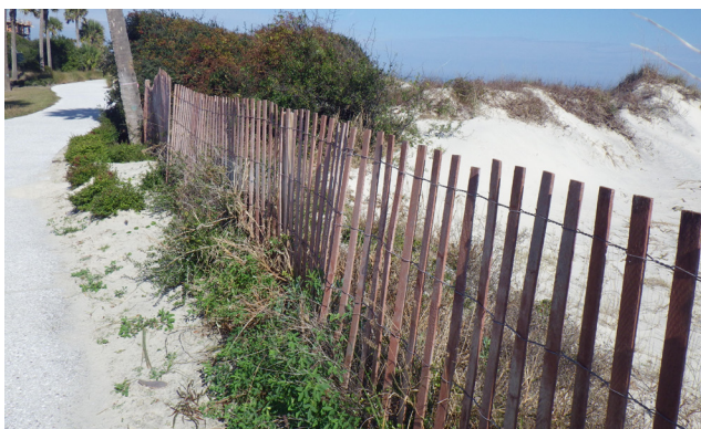
Figure 1. Sand Fence and Native Plants
