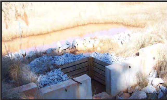
Example of Slotted Board Dam
