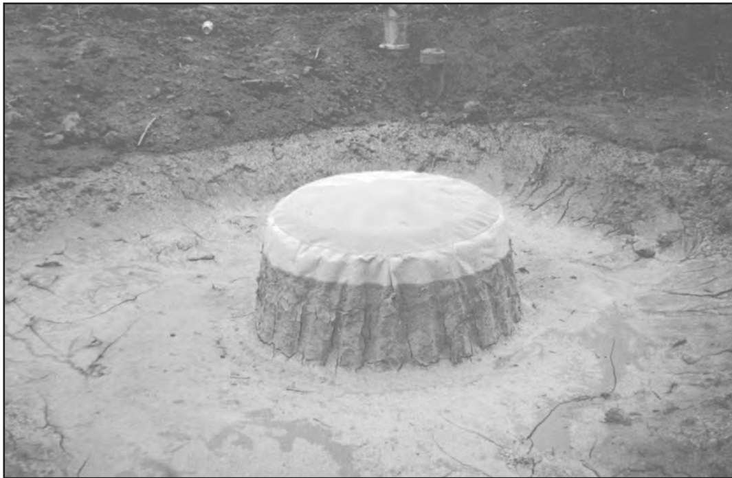
Figure 6-28.7 Equivalent Inlet Sediment Trap
