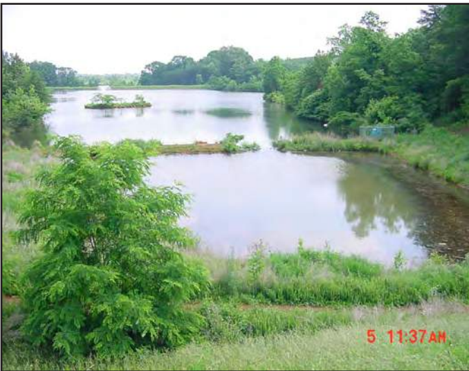
Post-construction conversion called for the creation of sediment forebay in this larger scale pond.
