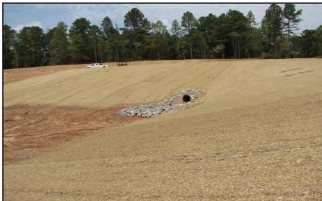
Figure 2.8 - Matting can assist in rapid establishment of vegetation.
