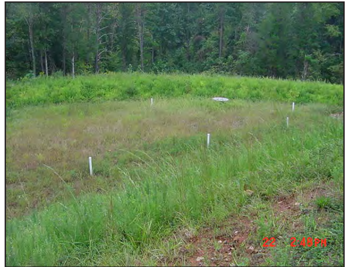
Conversion of a sediment basin to a bioretention area. The original riser acts as the overflow structure for the bioretention practice.
