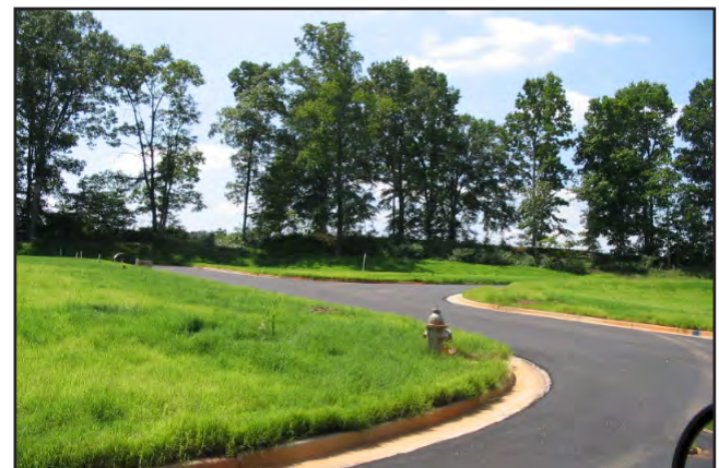
Figure 2.6 - Vegetation on this road bank will reduce erosion to a minimum.
