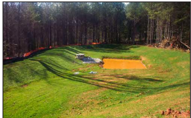
Figure 2.10 - Storm water detention structures will reduce storm water runoff from developed areas.
