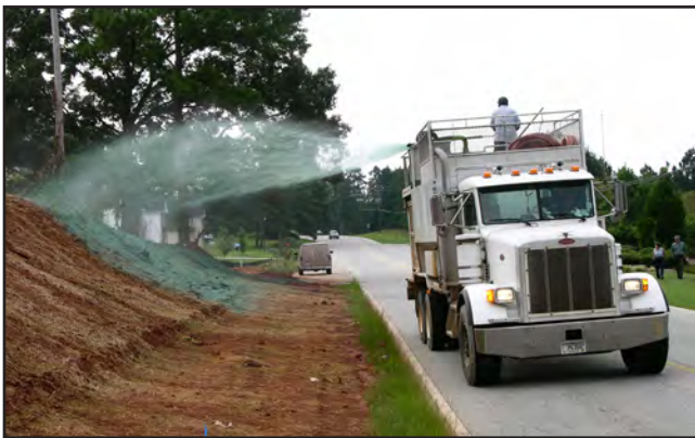
Figure 2.7 - Hydroseeding equipment can efficiently and quickly establish disturbed areas.
