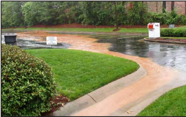
Figure 2.13 - Offsite impact from a neighboring construction site.
