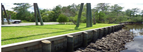
Rip Rap Bank
