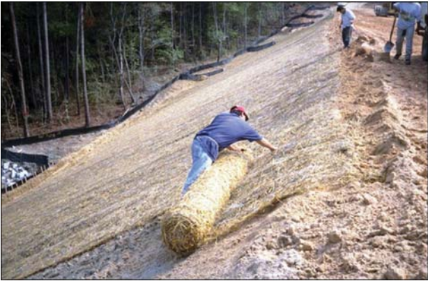
Figure 2. Installation of Jute Matting
