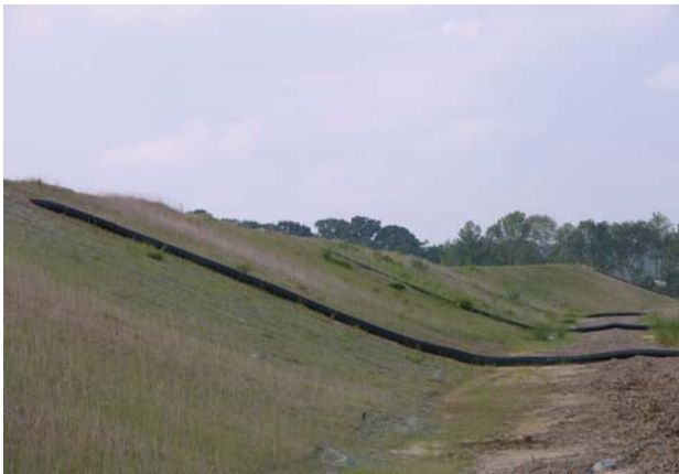
Figure 2. Diagonally Placed Downdrain
