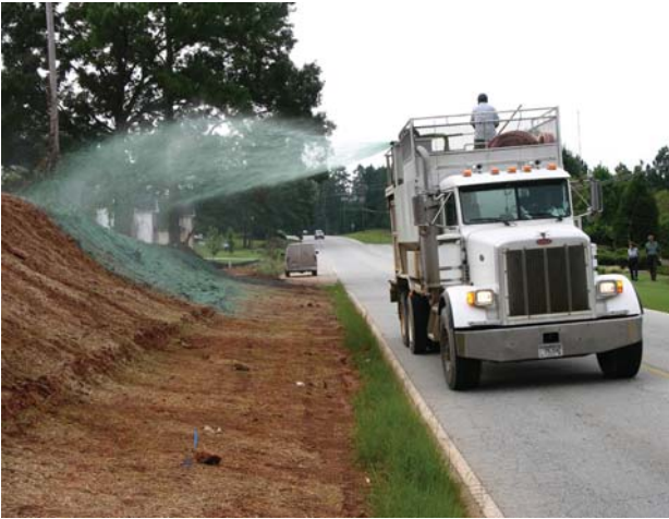
Figure 1. Hydroseeding on disturbed areas
